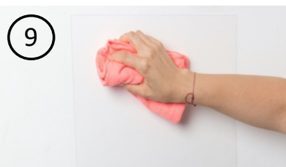
9 Using a rag and side-to-side motion to avoid air bubbles forming.
