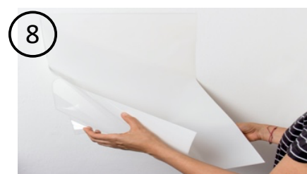
8 Carefully remove the remaining liner, while attaching the film to surface.
